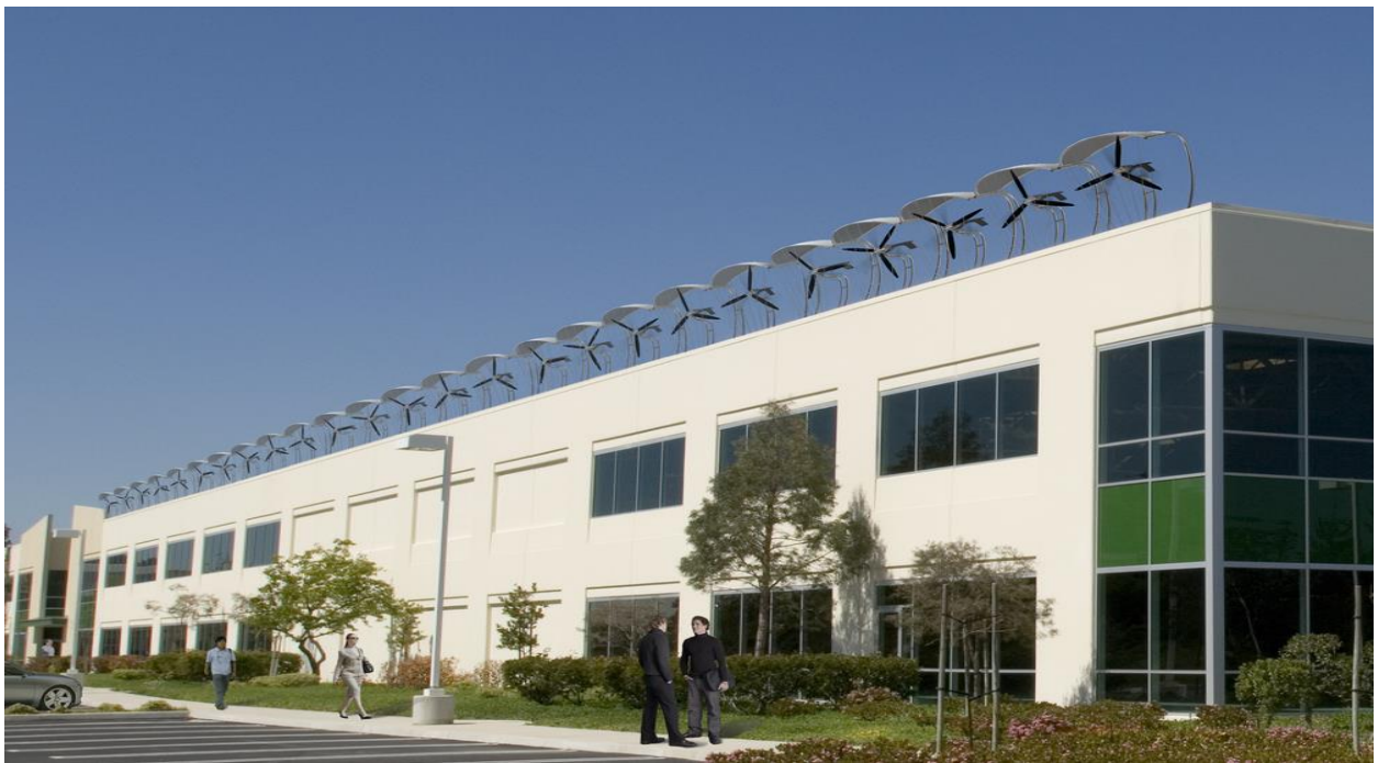
Illustration 5. Micro wind turbines that are integrated into the building infrastructure (ClimateTechWiki, 2018).
