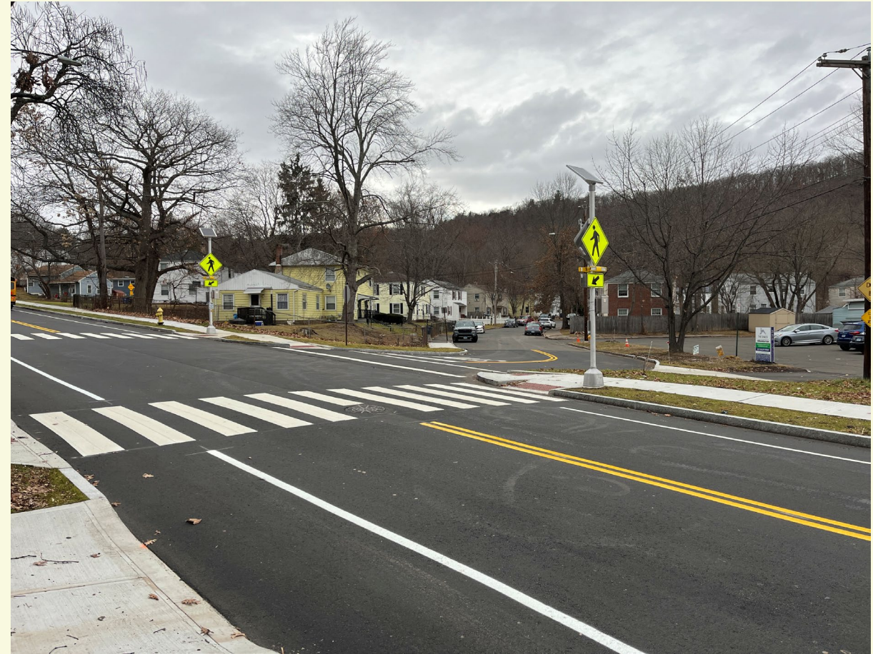
Crosswalk with RRFB (rectangular rapid flashing beacon)
